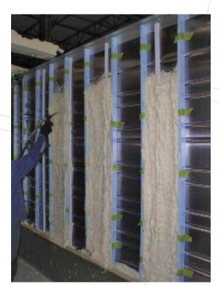
The Touch 'n Seal Refill System is a Class I, fire retardant, high performance spray polyurethane foam dispensing system for both new assembly and repair of all types of transport vehicles. Use Touch 'n Seal Refill Systems to repair, insulate and provide structural strengthening for trailers, vans, reefer bodies, emergency response vehicles, buses, aircraft and personal watercraft. Touch 'n Seal Refill Systems also provide exceptional sound and vibration reduction in all types of structures.
